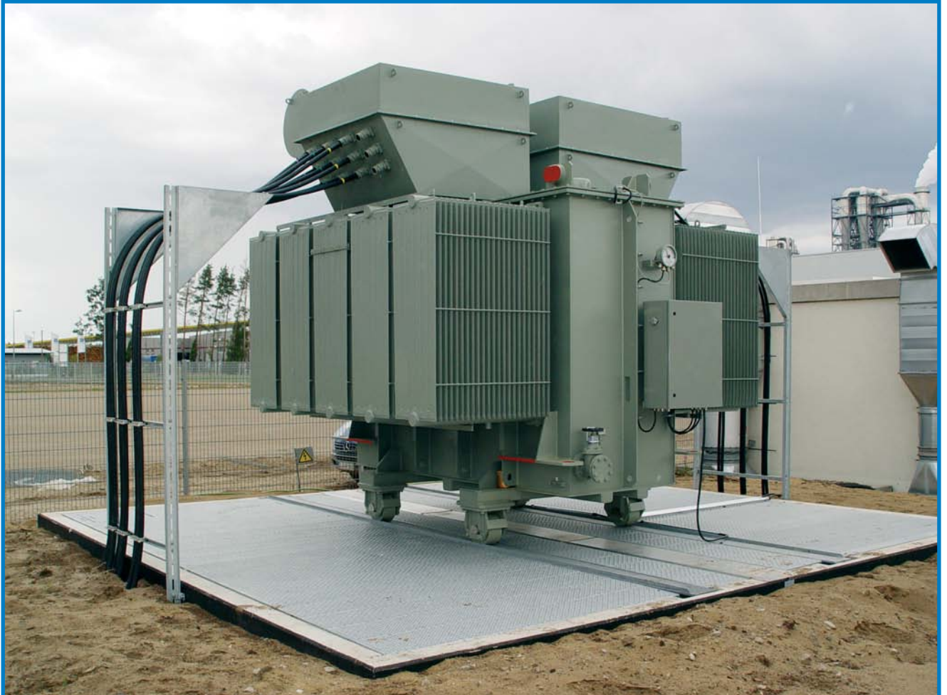
20 MVA-Transformator 20 kV/10 kV ▲
